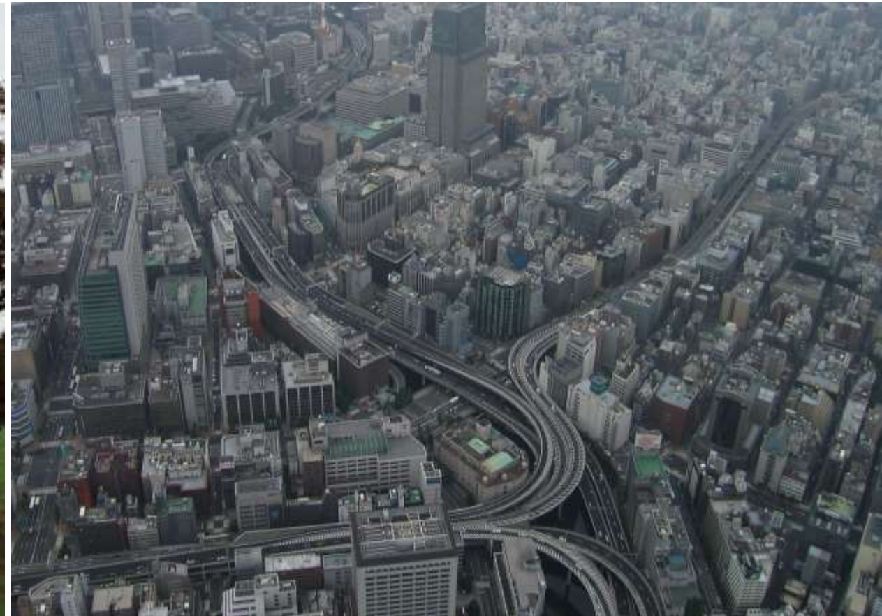
Metropolitan Expressway in Tokyo
